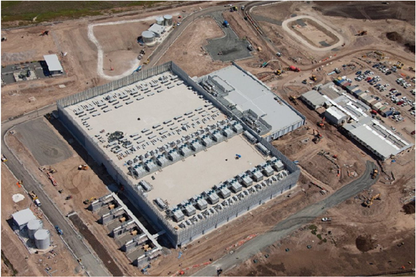
FIGURE 25.11 Aerial view of (42) indirect air-side economizers (IASEs).
